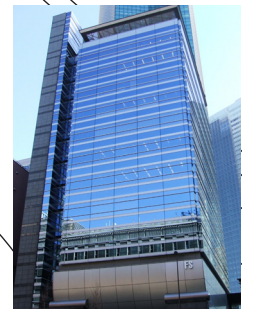
FSビル FS Building
